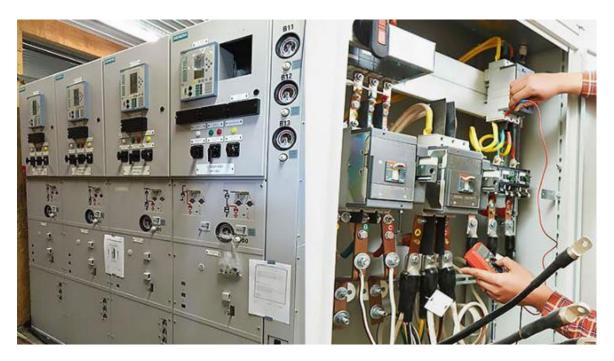
As you may know, the main function of a switchgear is to receive electricity and distribute in to circuits within a buildings. Switchgears must be designed and manufactures in a way that (1) properly controls the current and (2) provides proper protection. In addition, a switchgear should be able to detect the size and intensity of fault and isolate the faulty section from the whole system within the shortest time possible.
