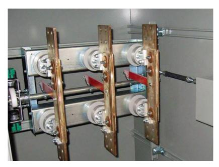
Knife switches are used in MV switchgears when isolation is needed to separate certain parts of switchgear for maintenance or other works like grounding. They are operated manually under no-load condition and using motors and compressed air for remote control mode. The size of these switches should also be considered when designing switchgears.
